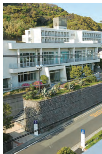
研修棟外観 Appearance of Building for In-service Training
